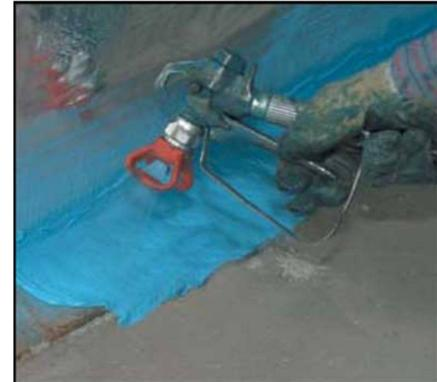
Figure 6. Applying smoke sealant.
