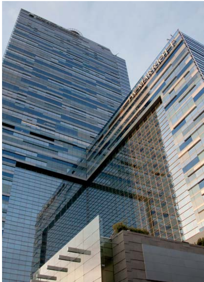
Thermafiber® TopStop® Head-of-Wall insulation contributes to energy conservation and fire protection in the LA LIVE complex in Los Angeles, CA.
