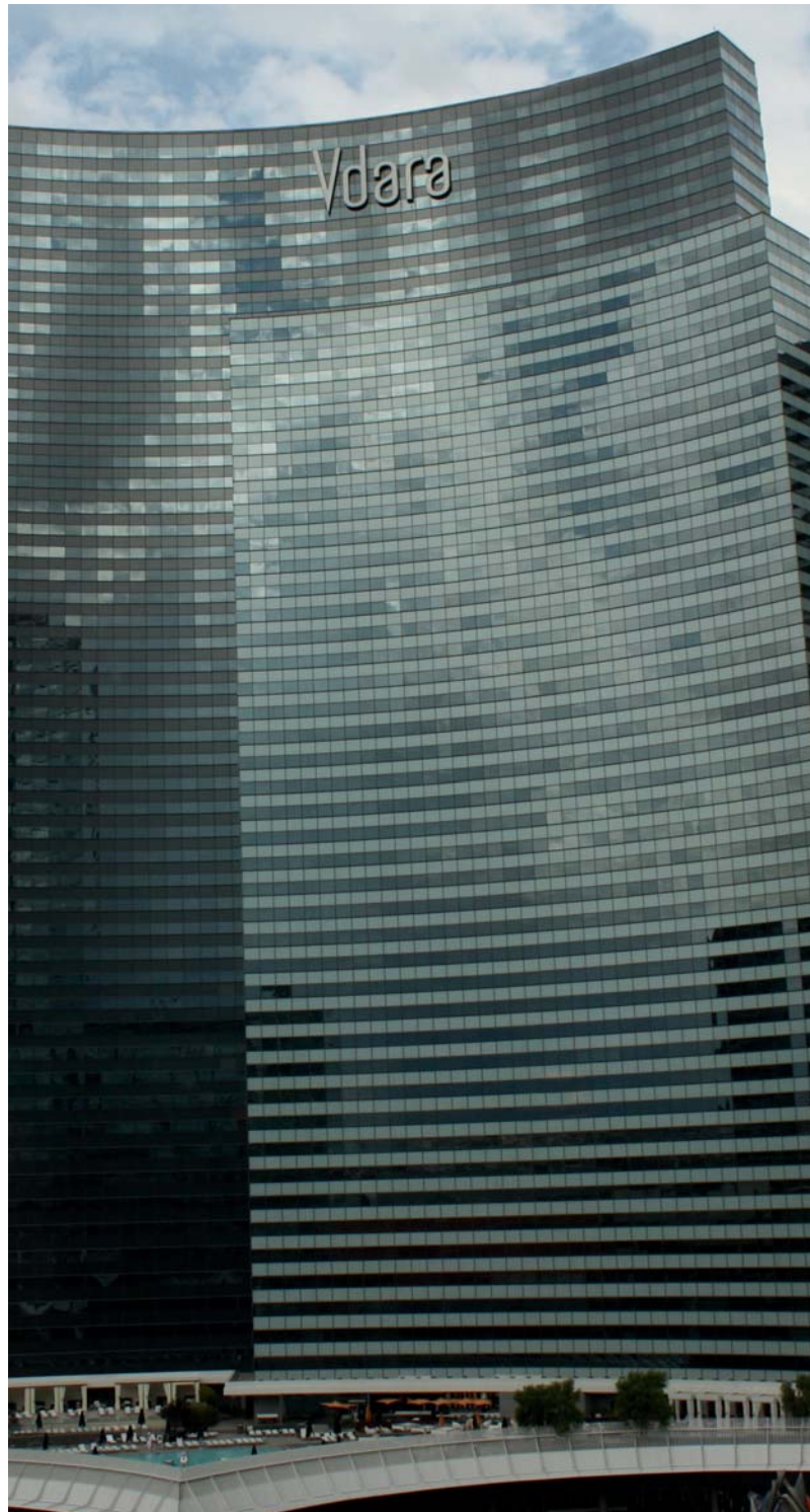
Spiral Anchors in conjunction with Thermafiber ® Impasse ® Insulation Hangers were used in the perimeter fire containment system in the Vdara Hotel in Las Vegas, NV.
