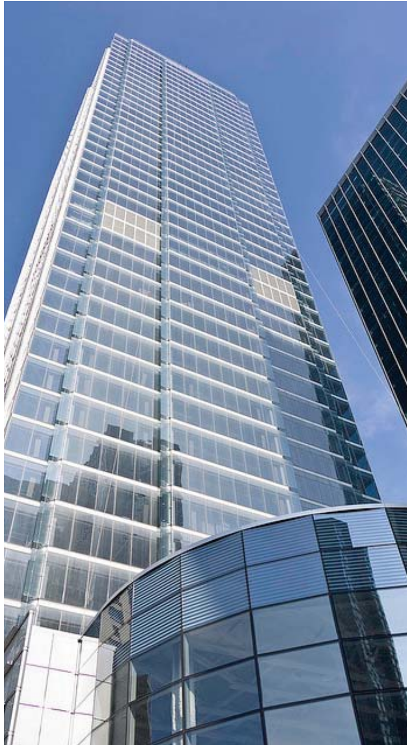
The Thermafiber® Impasse® Insulation Hanger System was used to install various Thermafiber® mineral wool products in the perimeter fire containment system at 353 N. Clark in Chicago, IL. Thermafiber® mineral wool insulation contributed to this building's LEED® Gold status.
